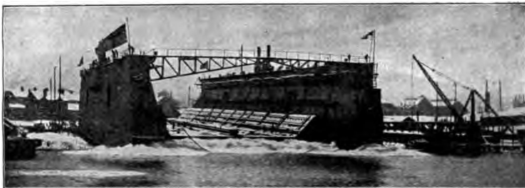
LAUNCHING A GREAT FLOATING DOCK.
